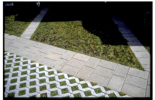
This option can be easy to install and maintain, cost-effective, and can add aesthetic value to your project. Permeable pavements may include pervious concrete, pervious asphalt, porous pavers, crushed aggregate, open pavers with grass or plantings, open pavers with gravel, or solid pavers.
